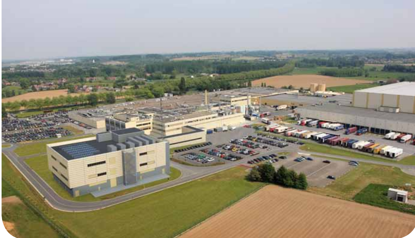
Baxter in Belgium – Production site in Lessines
